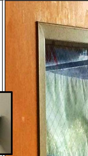
The thickness of the molding is typically 1/16 to 1/4 inch for steel or aluminum moldings and about 3/8 inch to 3/4 inch for wood moldings. This measurement is to assure proper spacers are included with the shutter. Do not measure molding depth from glass.
