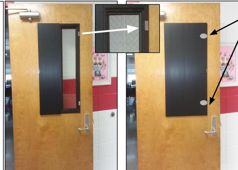
Magnets are inside the material and only a half inch from the working edge. Our steel adhesive plates need to align with the magnets if the molding is not made of steel.
