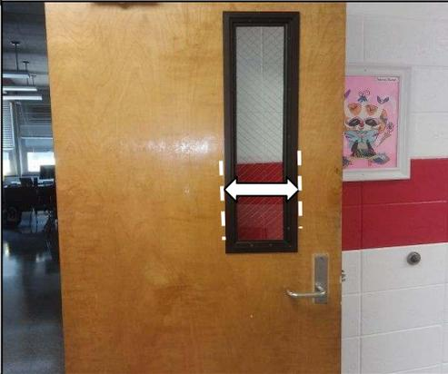
Measure width from outside edge to outside edge of the raised molding around the window
