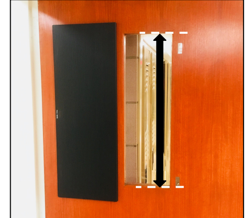
Measure length of the glass from top to bottom.
